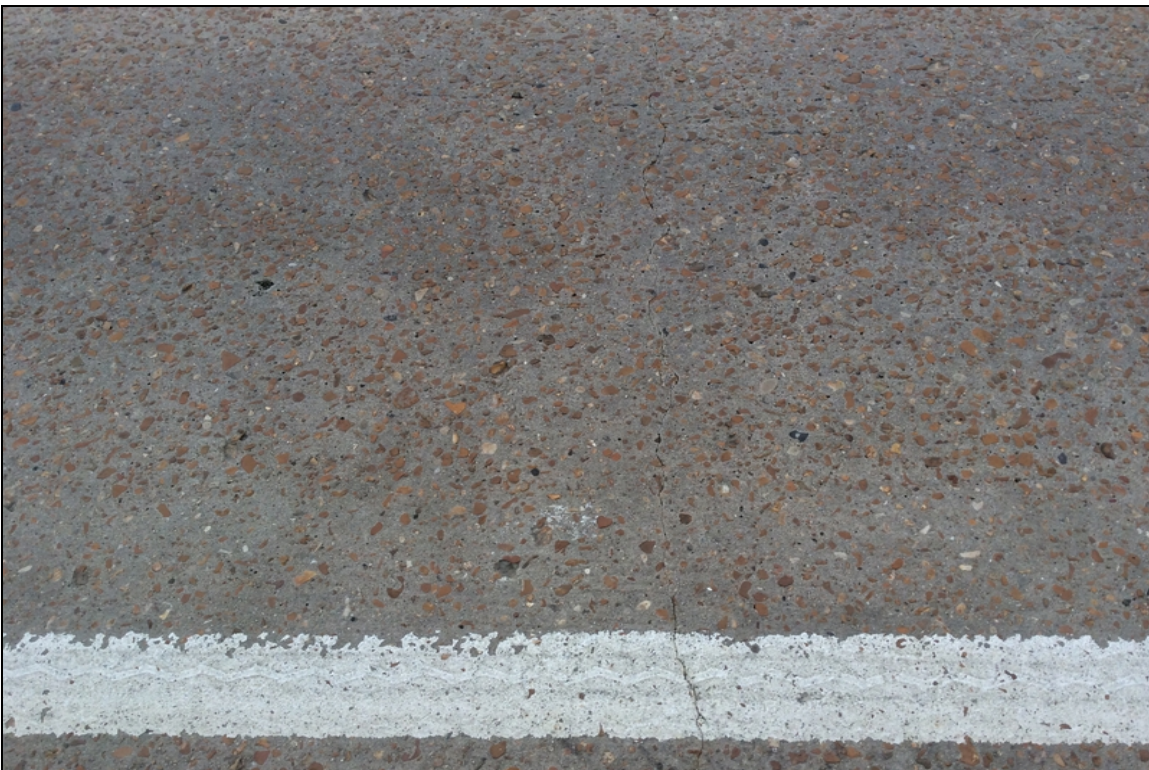
Typical cracks to deck @ all spans
