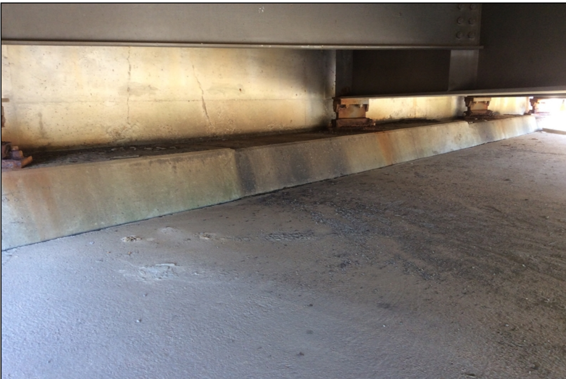
Typical cracks to Abutment 1 & 2.
