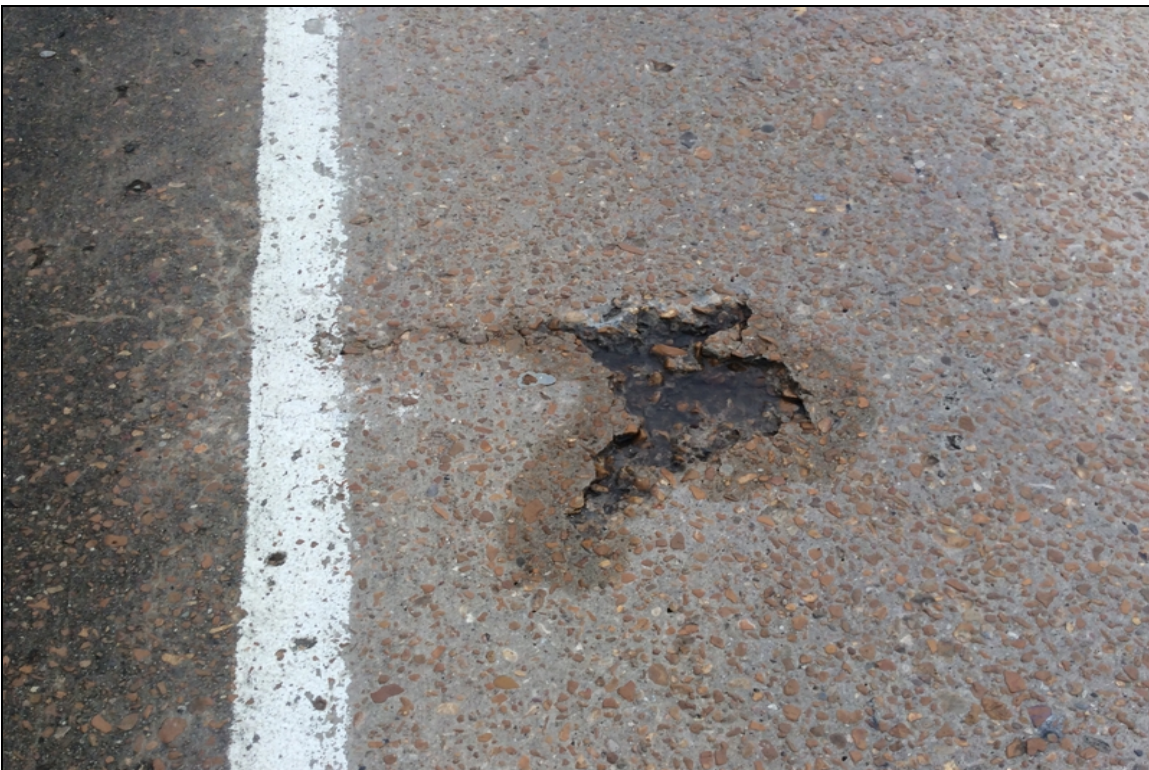
Spall to deck @ Lt side span 1.
