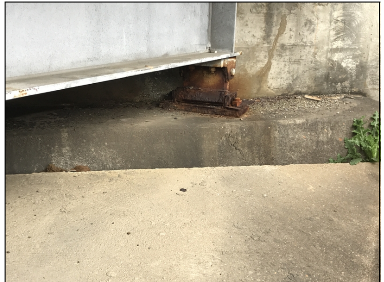
Rust & corrosion to bearings @ Abutment 1 & 2.
