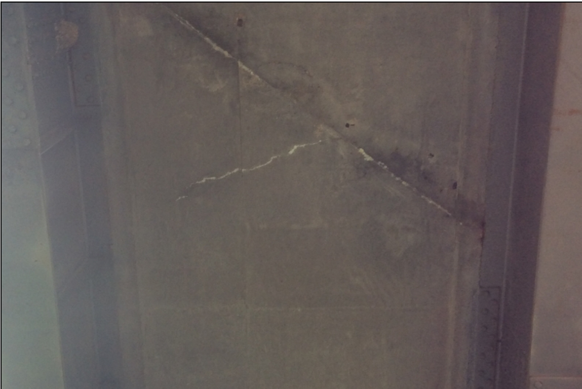
Typical efflor cracking to deck @ all spans
