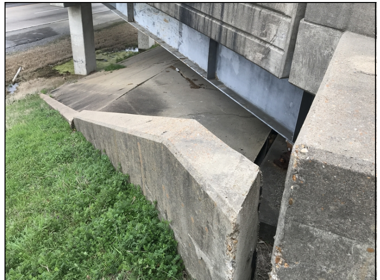
Concrete rip rap has settled, cracked & separated @ Abutment 2. Also Rt wing @ abutment 2 is separated.
