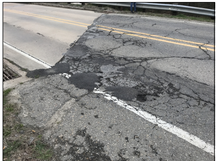
Roadway settled & uneven @ Abutment 1 & 2.
