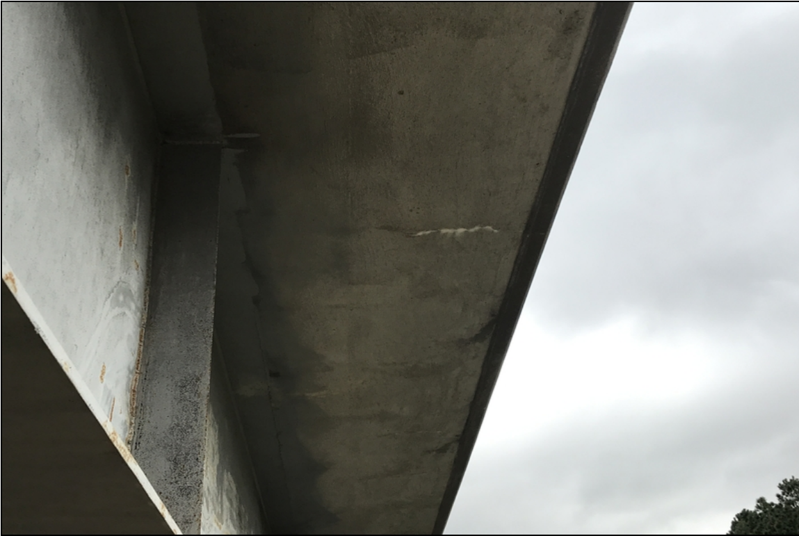
Typical efflor cracking to Lt and Rt overhangs.
