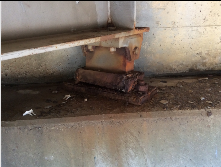
Rust & corrosion to bearings @ Abutment 1 & 2.
