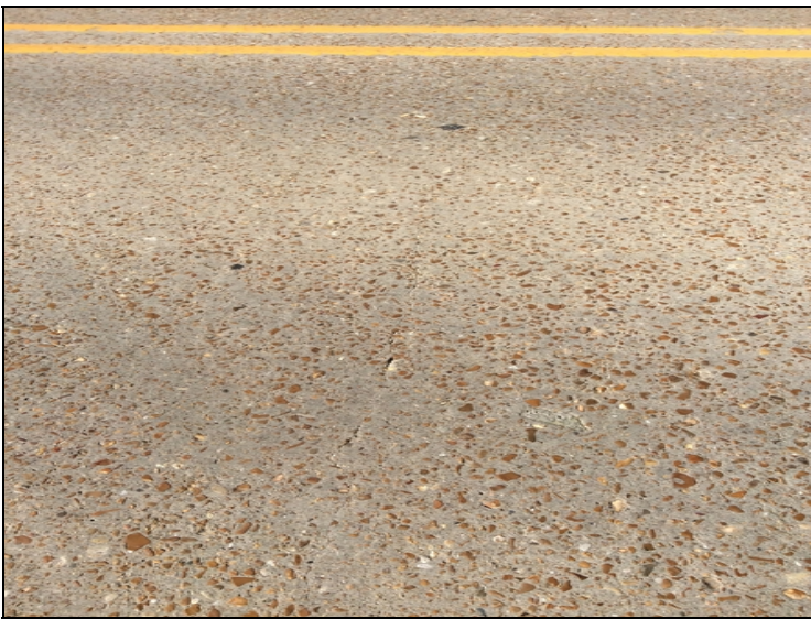
Unsealed cracks to deck @ all spans & approach slabs @ Abutment 1.
