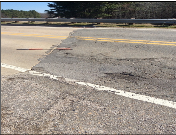
Roadway settled & uneven @ Abutment 1 & 2.
