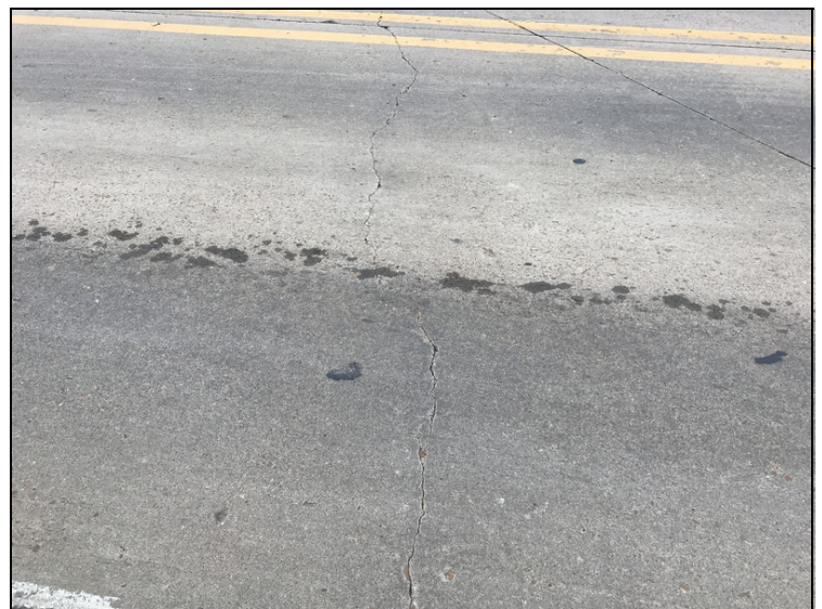
Unsealed cracks to deck @ all spans & approach slabs @ Abutment 1.
