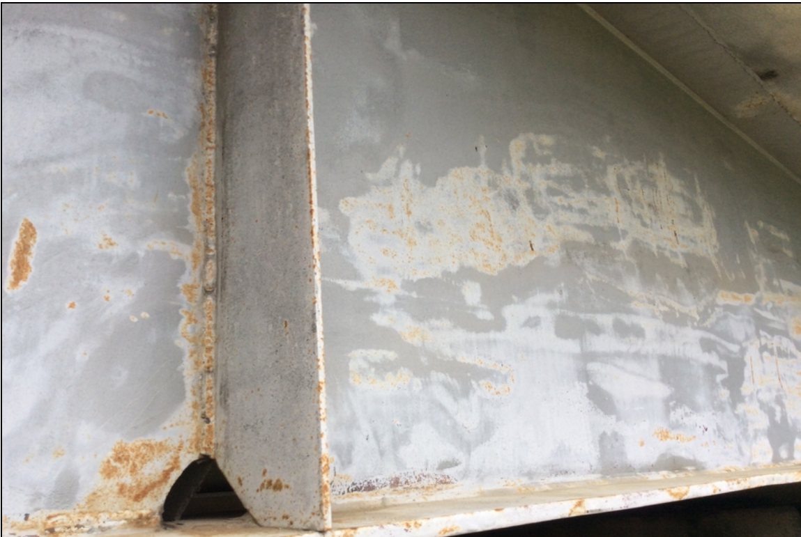
Areas of rust & corrosion to girders.
