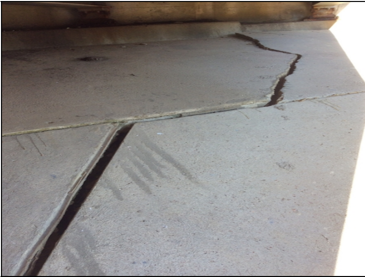
Concrete rip rap has settled, cracked & separated @ Abutment 2.
