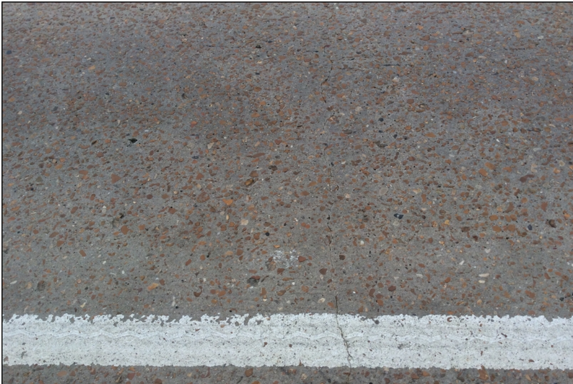
Typical cracks to deck @ all spans
